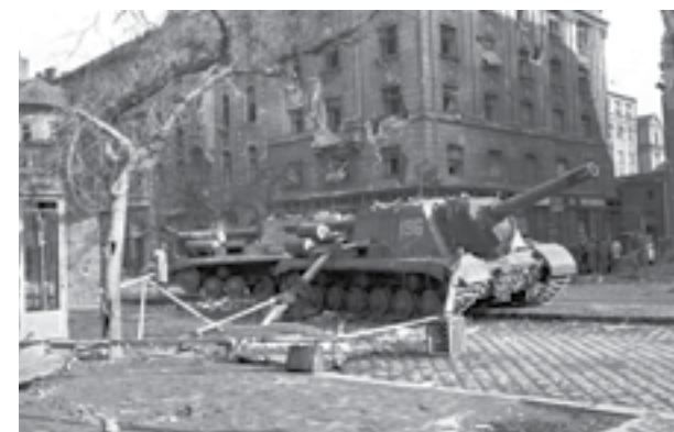
Destroyed buildings in Budapest. 1956. Fortepan / Berkó Pál
