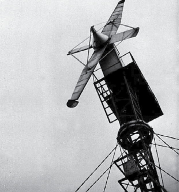
The Gedser wind turbine, designed by Johannes Juul in 1957, is significant in the development of modern turbine technology. It fed directly into the grid, and many of the elements still feature in contemporary turbines. NASA studied it in 1975 as the U.S. looked to build their own wind energy capacity. © Electricity Museum, Bjerringbro.
