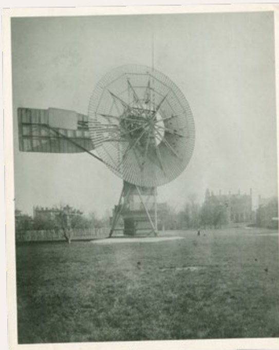
Charles Brush's 1888 wind turbine, capable of supplying enough electricity for most of the lights and motors in his home for 20 years. It was 60 feet tall and weighed about 80,000 pounds. Image courtesy of The Western Reserve Historical Society, Cleveland, Ohio.
