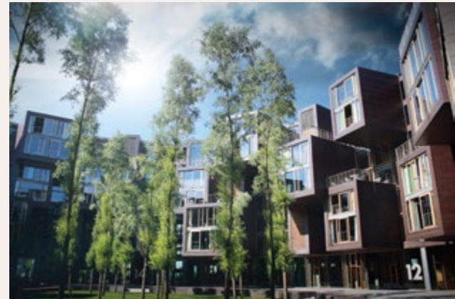
Crowne Plaza Copenhagen Towers was given the 2010 EcoTourism Award. Some of its technologies include having 2000 m 2 of solar cells (the largest building-integrated installation in Northern Europe) and the first groundwater-based heating and cooling plant in Denmark. It is also carbon dioxide neutral. © State of Green.
