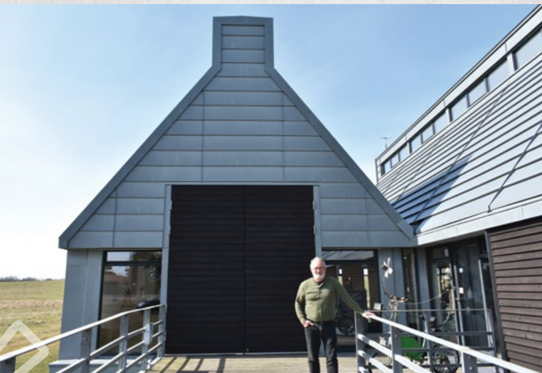
Søren Hermansen, Director, outside of the Energy Academy. The building is designed to maximize efficiency, from using natural ventilation and passive solar heating, to rainwater for toilets. Image courtesy of Diya Nagaraj.
